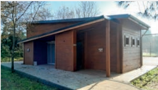
Postane mahallesi-Mercan park Wc
